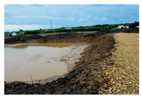
How many of you remember this picture, taken in May of 2008? The foundation of this building had just been dug and a heavy rain turned it into a manmade lake. The problem stemmed from the fact that our land was mostly a mucky clay which not only holds in water but also makes for a very poor foundation. As a result, the estimated cost for our foundation doubled in price. The
